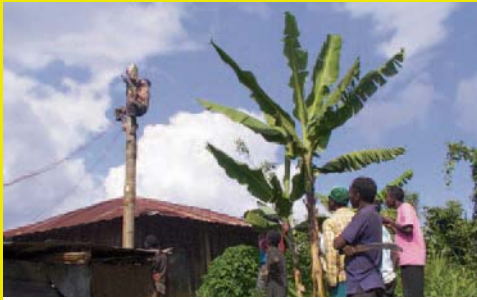
Installation of electric posts in Kathamba.
