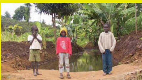
Installation of the water reservoir in Kathamba.
