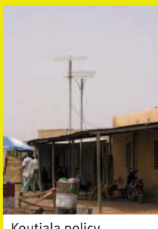
Koutiala police station electrified by the ESCO.
