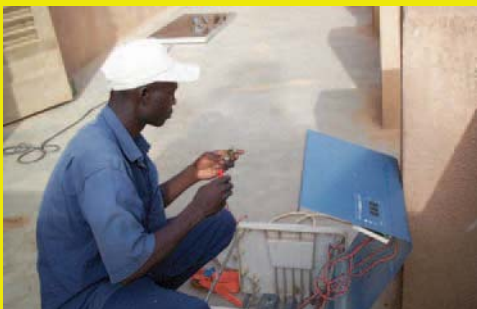
Preparation of a battery box in the ESCO office.
